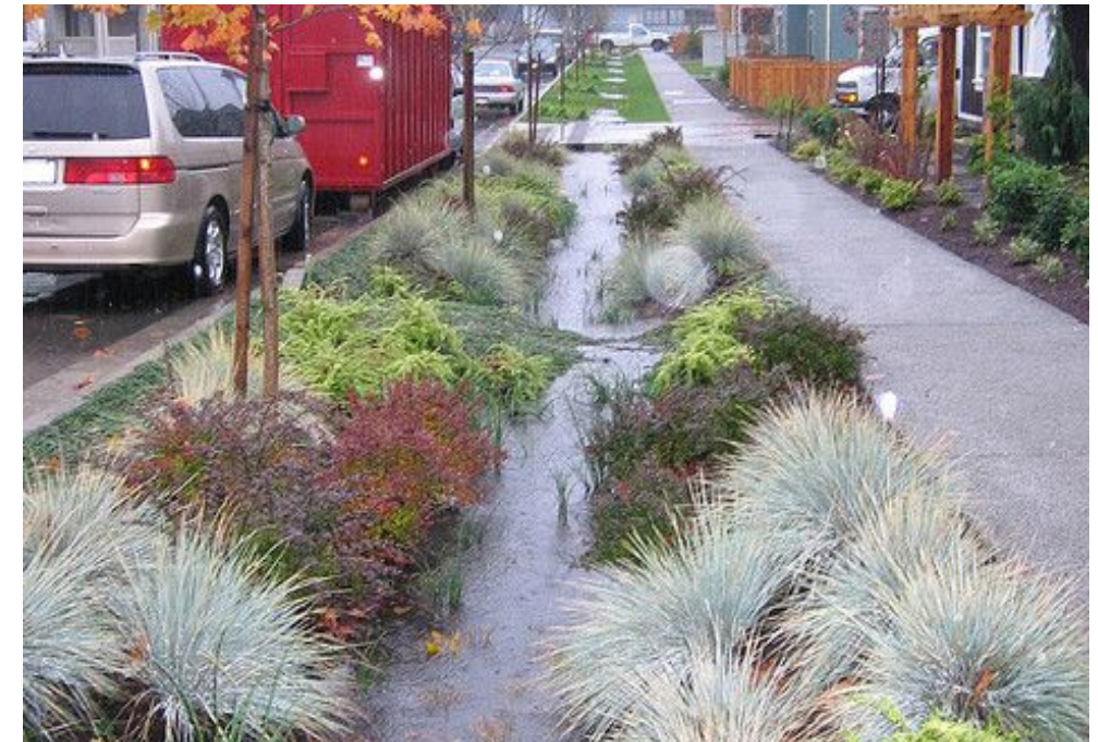
Rain water garden
