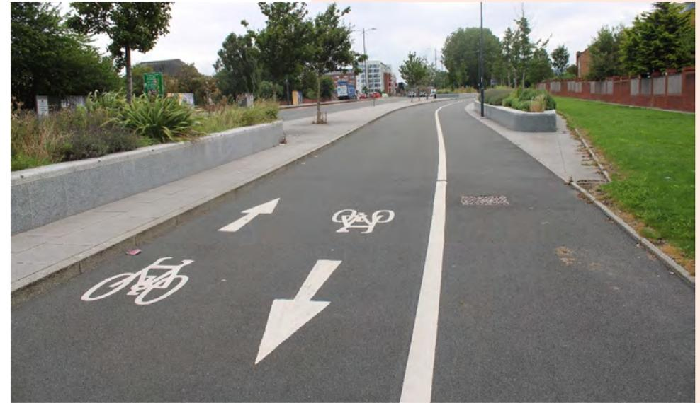
**Figure 3.2: Separated cycleway with floating parking bays, Duke Street, Birkenhead**
