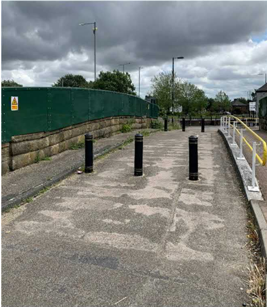
Figure 3-30 - Bollards preventing vehicles accessing this road
