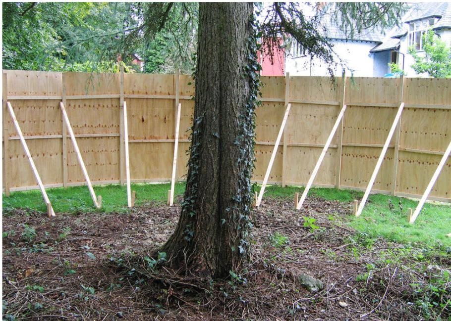
**Picture 5.4 Close board fencing can also be used to secure tree protection areas.**
