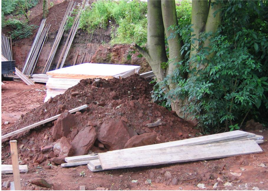
**Picture 5.1 Storing rubble, soil and other building materials will lead to compaction of roots and death of a tree.**
