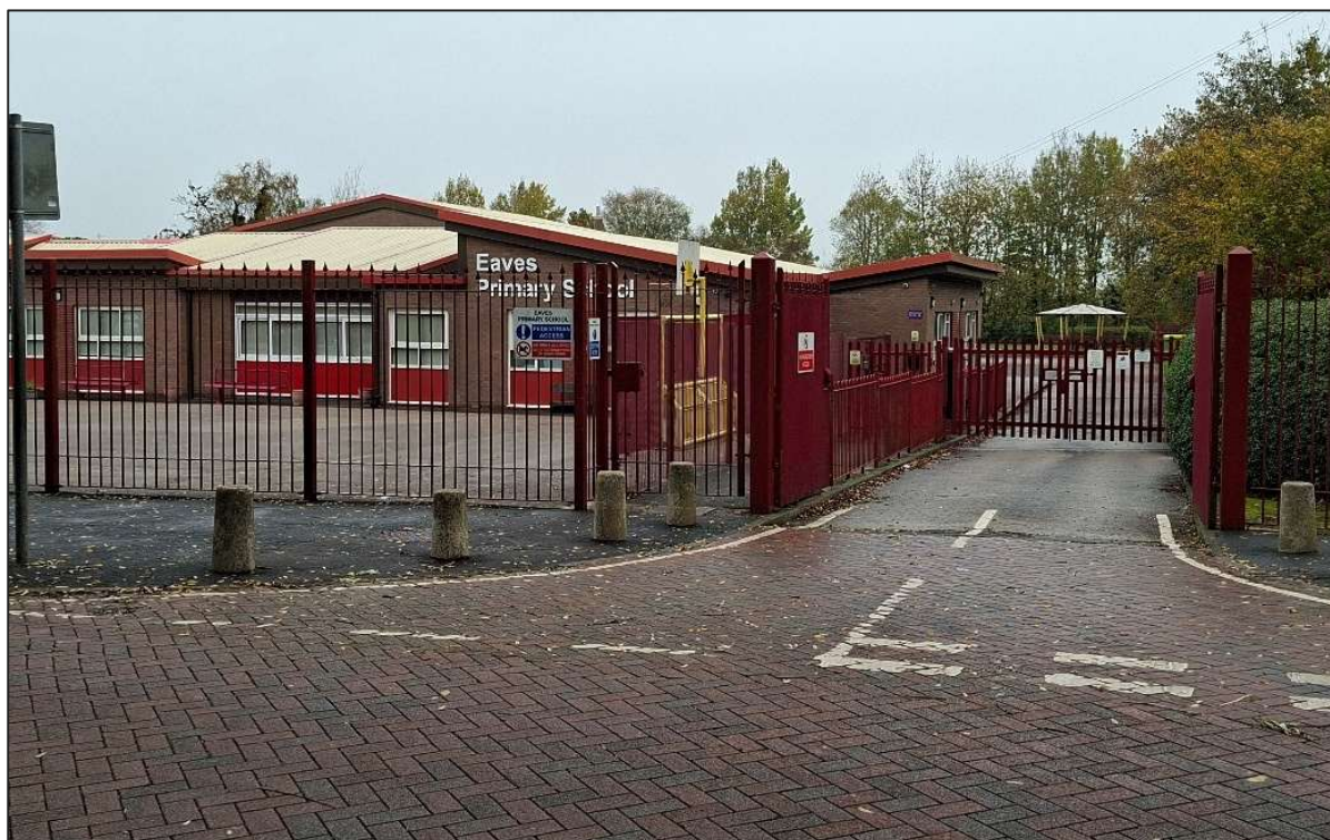
Figure 3.37: Eaves Lane – Eaves Primary School Pedestrian Access
