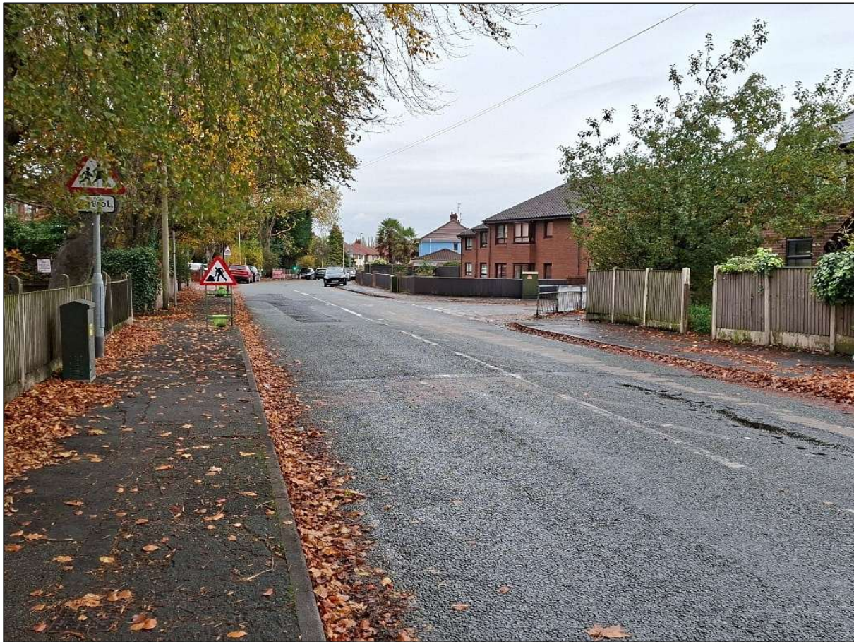
Figure 3.20: Leach Lane – Signage and Road Markings
