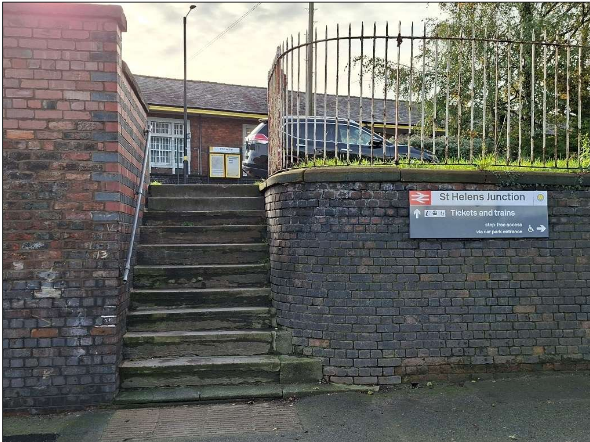
Figure 2.21: Station Road - St Helen's Junction Railway Station Stairwell Access
