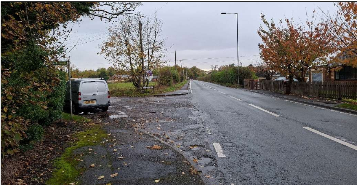
Figure 5.2: Gorsey Lane Junction
