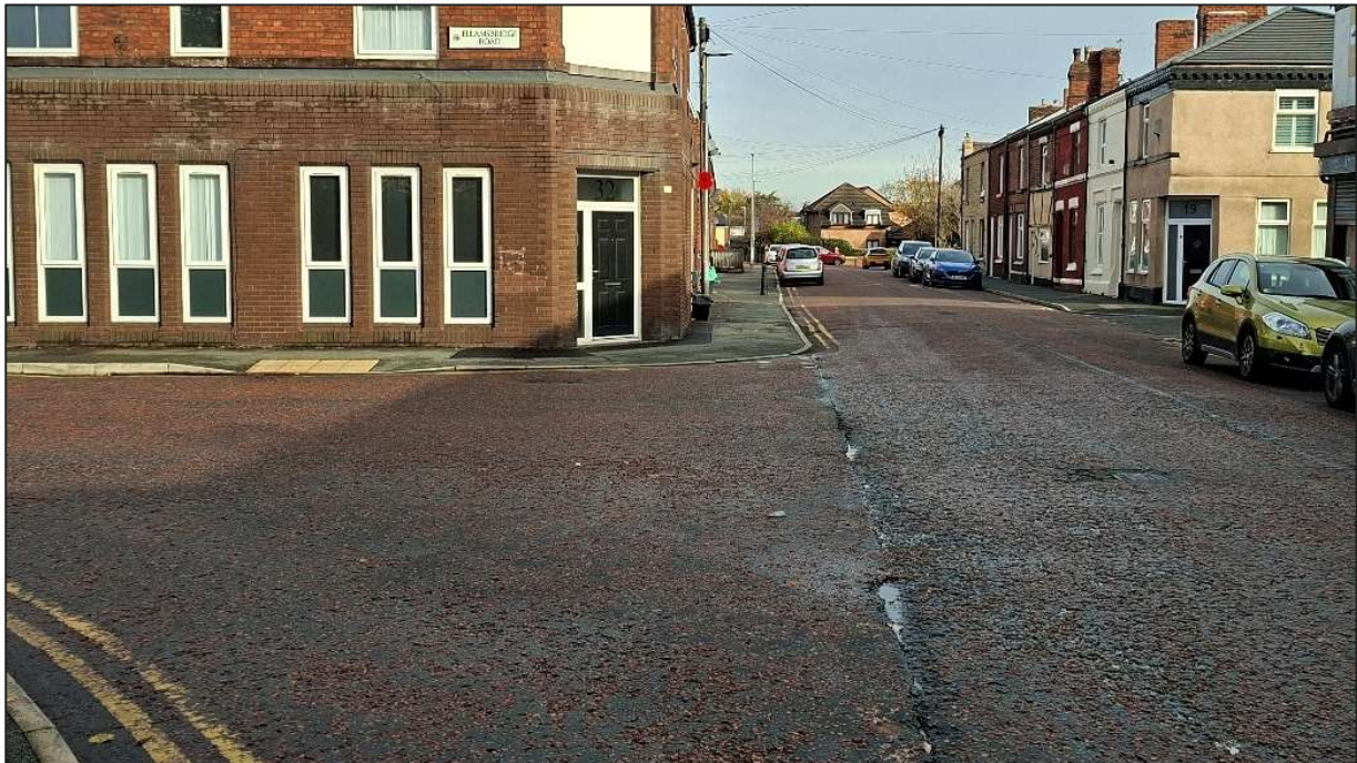
Figure 2.15: Junction with Ellamsbridge Road from Peckers Hill Road
