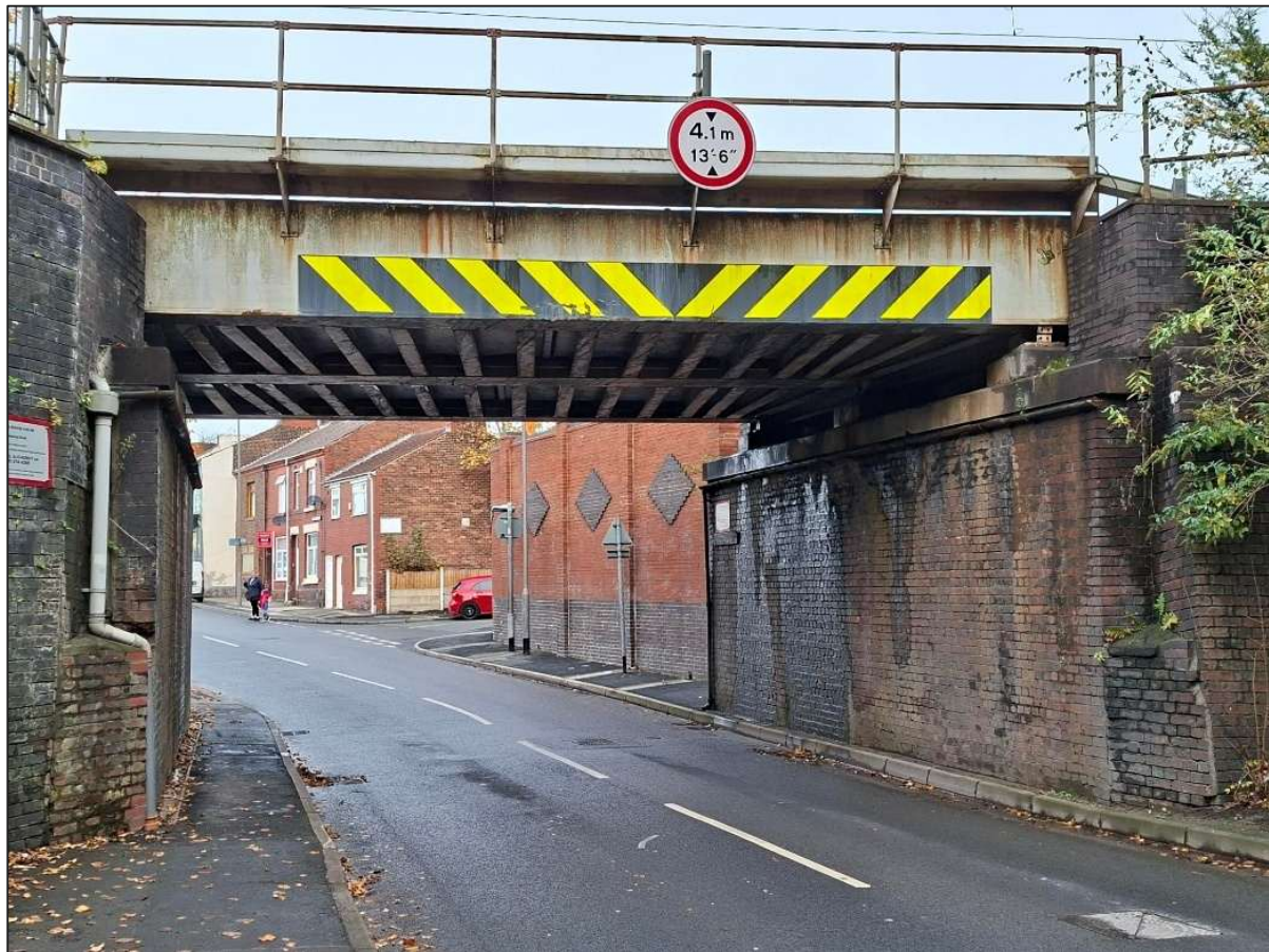
Figure 2.10: Helena Road - Underpass
