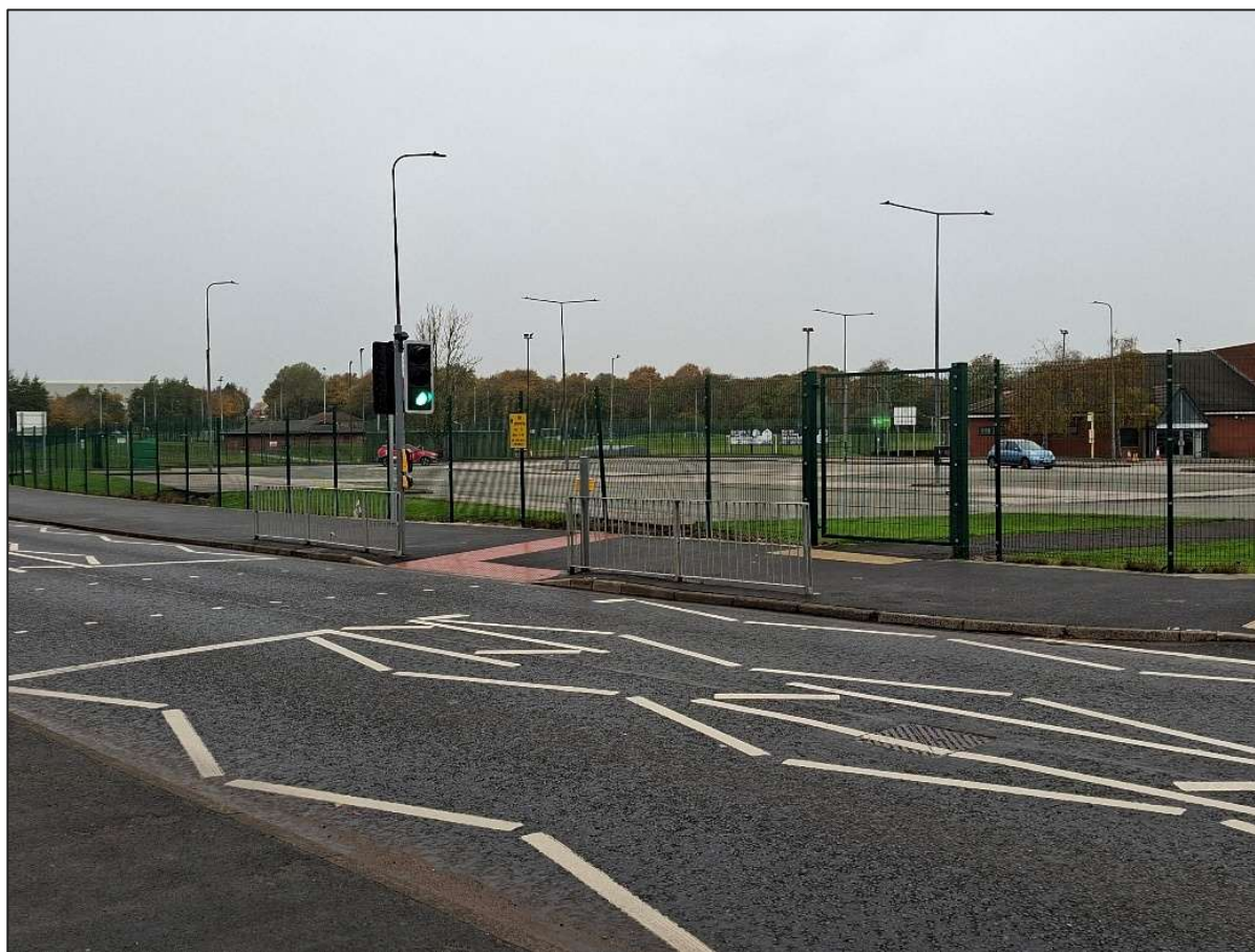
Figure 3.17: Sutton Leisure Centre Pedestrian Access
