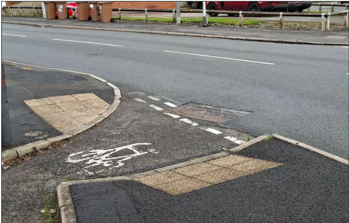
Figure 2.2: Cycle Access onto Helena Road
