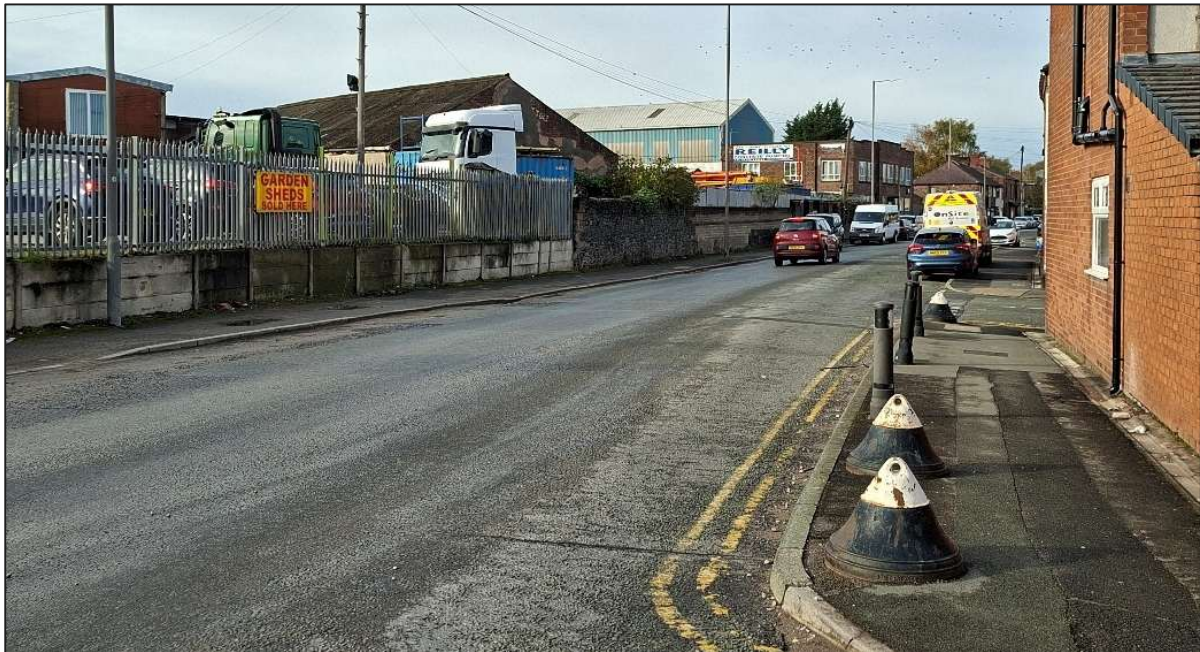
Figure 2.22: Station Road – Parking Bollards
