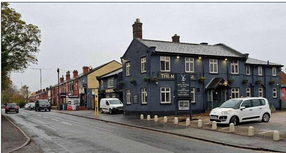
Figure 3.27: B5204 Mill Lane – Pub (The Millhouse)
