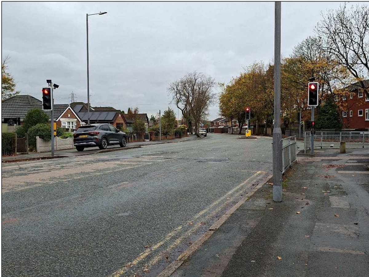
Figure 3.19: A569 Clock Face Road / Leach Lane
