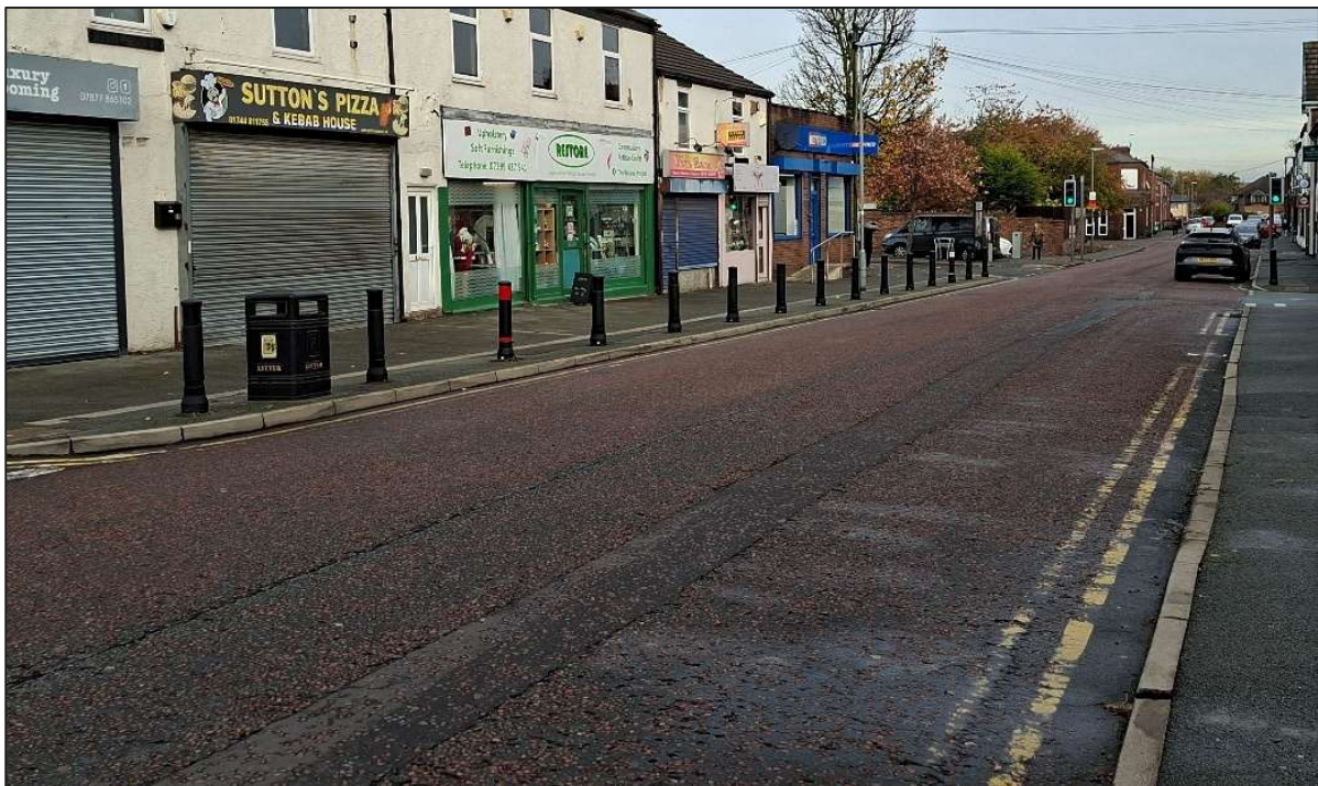
Figure 2.13: Peckers Hill Road - Pedestrian Bollards
