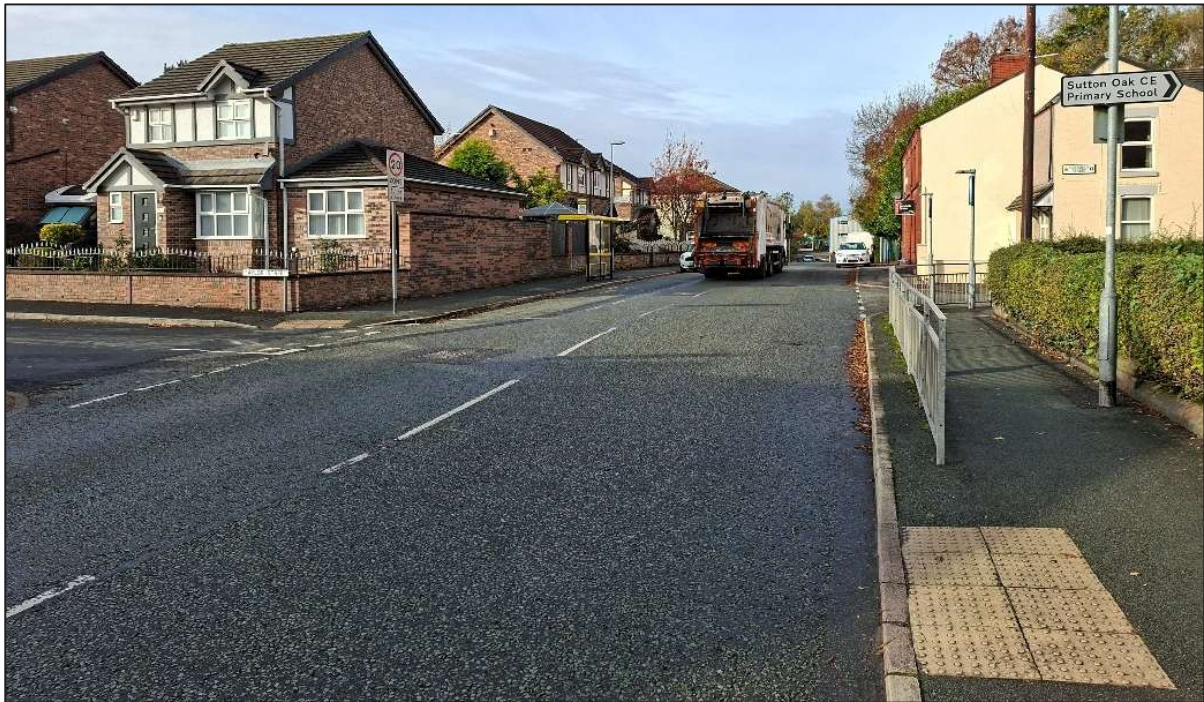
Figure 2.17: Ellamsbridge Road - Guard Railing
