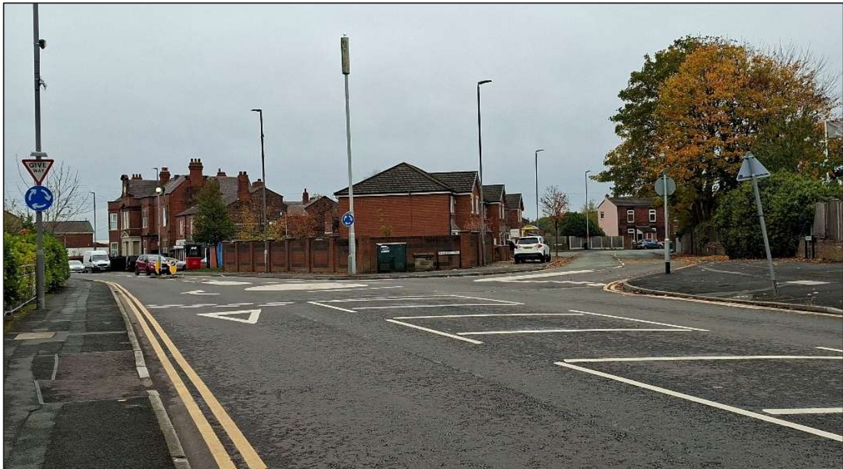
Figure 3.1: Clockface Road / Gartons Lane – Mini Roundabout Junction
