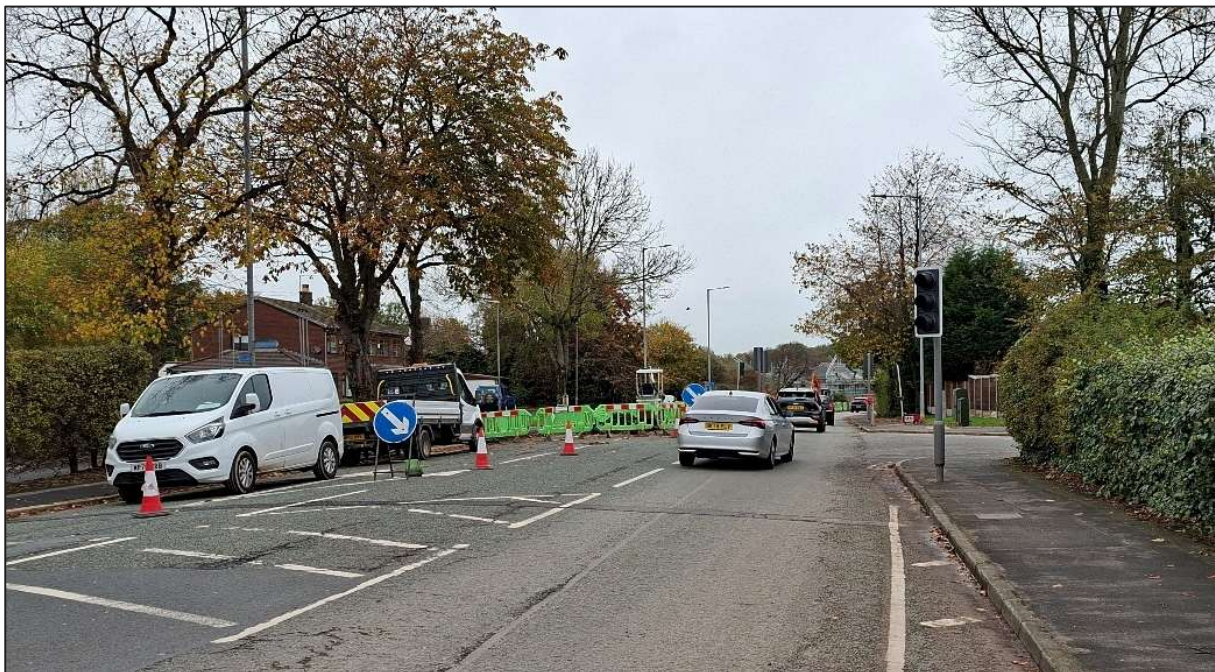
Figure 3.10: B5419 Chester Lane – Signalised Crossing
