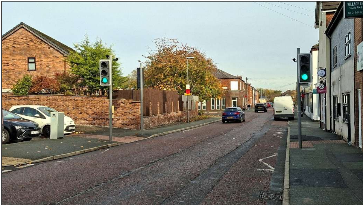
Figure 2.14: Peckers Hill Road - Pedestrian Crossing
