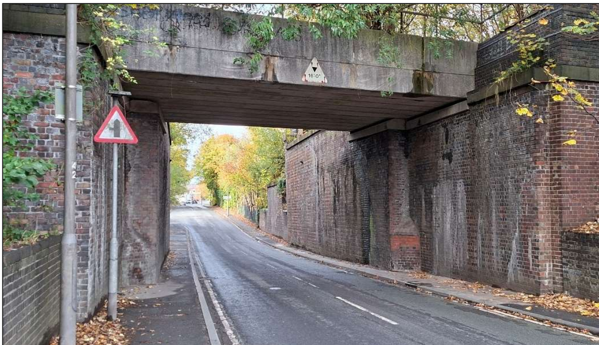
Figure 2.26: Underpass on Robins Lane
