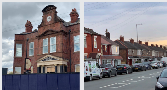
Former Clock Face PH (Clock Face Road) and examples of traditional worker's terraces (Reginald Road)
